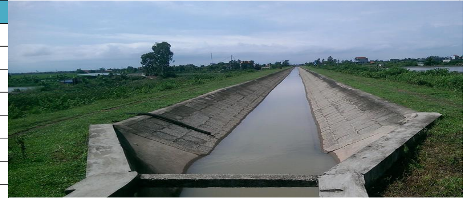
Reinforced canal section (Hai Nam island's segment)
