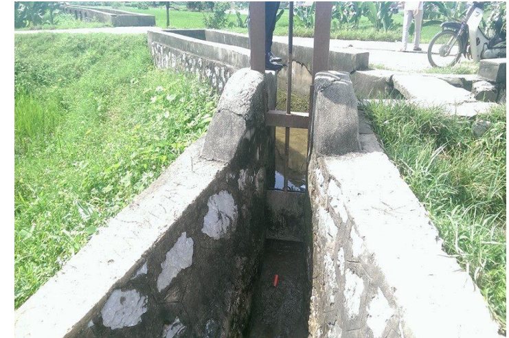
Intake at the beginning of 3rd level canal
