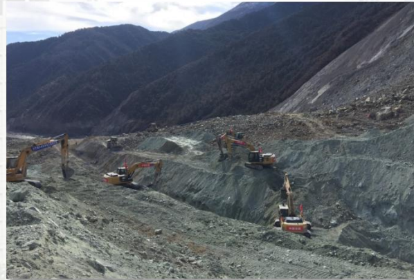
Excavation process of the spillway
