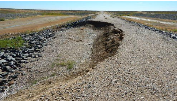
(b) Dam slope failure
