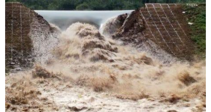
(a) Overtopping of dam failure
