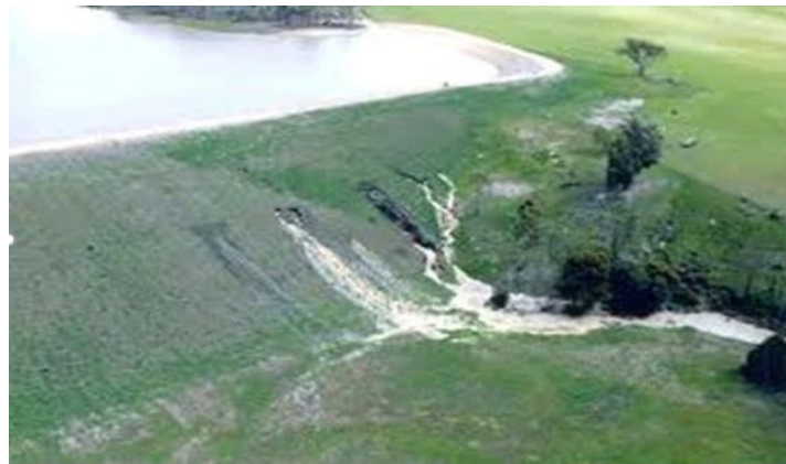
(c) Piping through dam body failure
