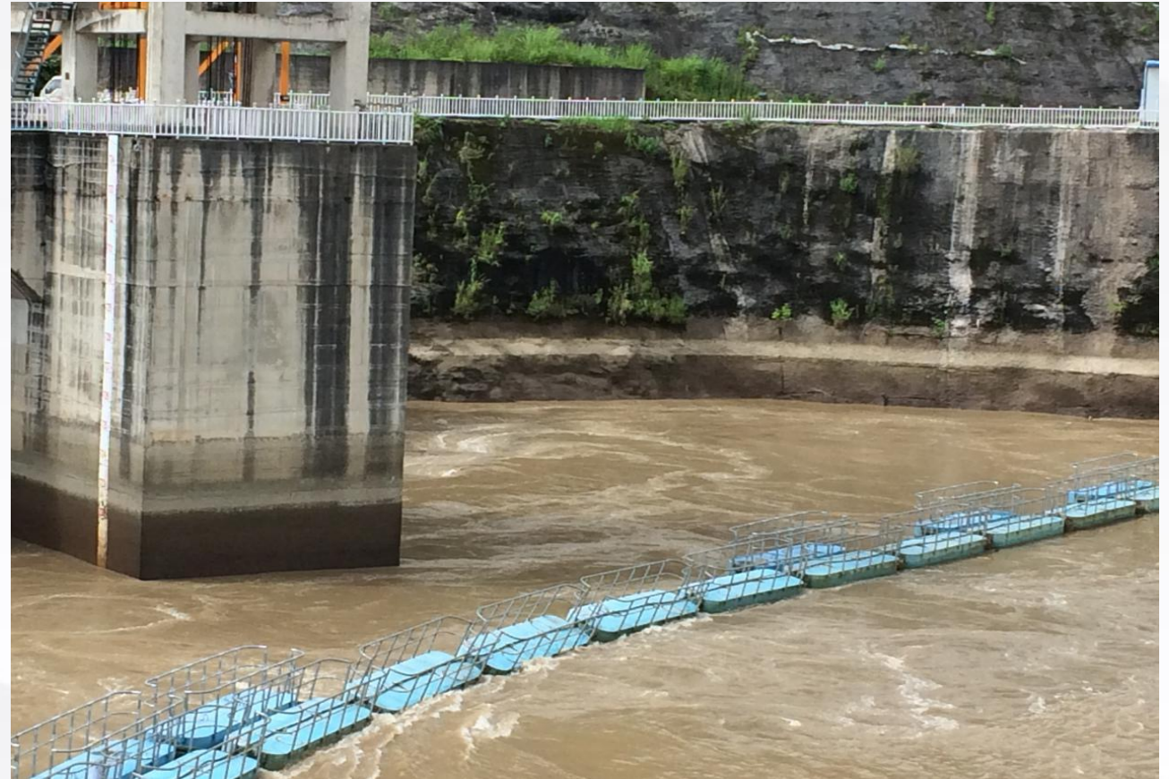
Floating-tank debris barrier tilted in operation
