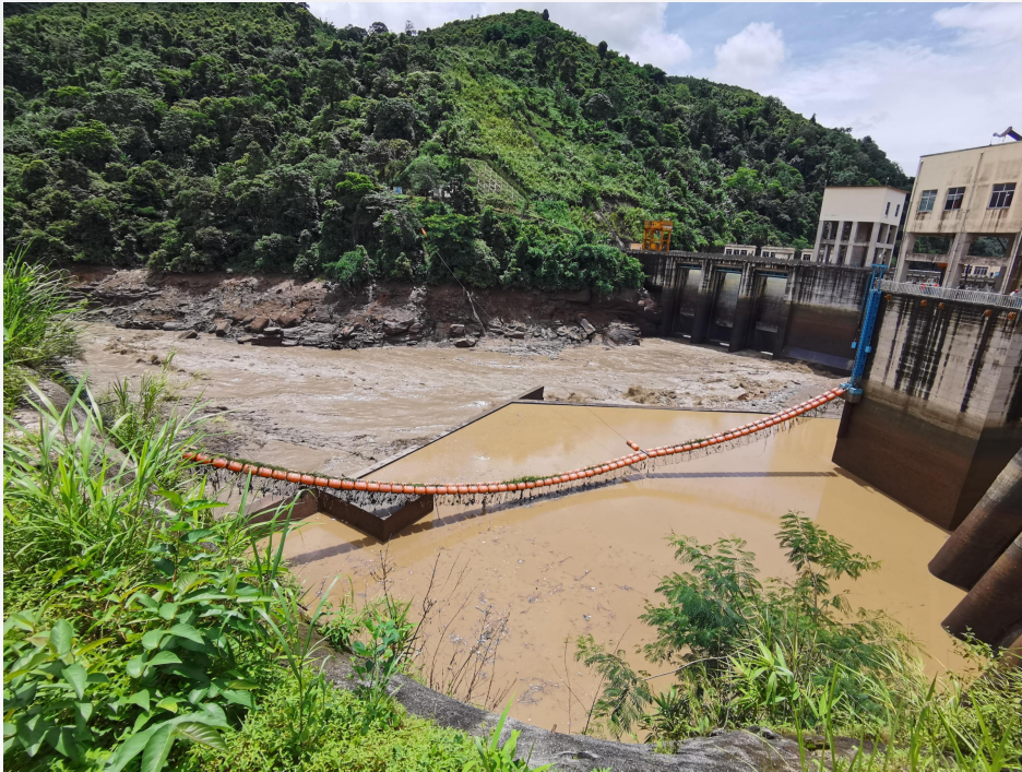
Independent hanging of the light-weight debris barrier
