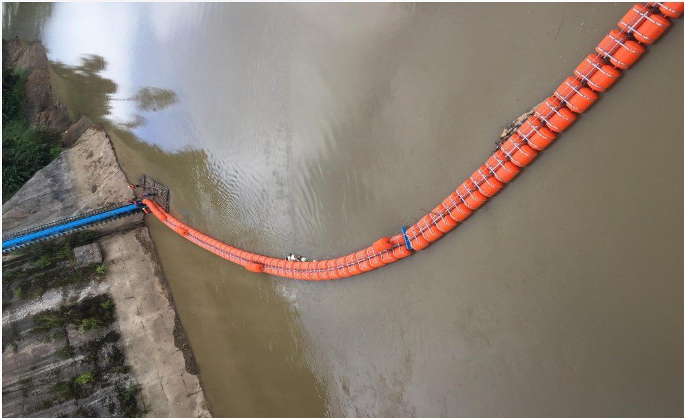
Modified as light-weight debris barrier
