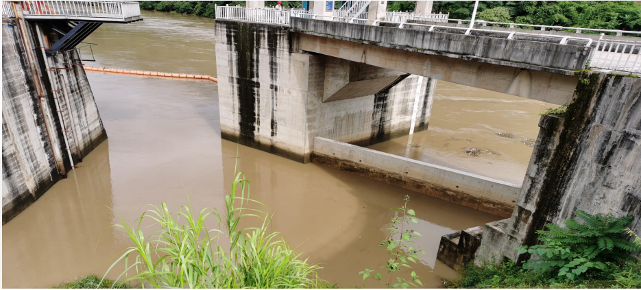
Stable retaining wall during sand flushing
